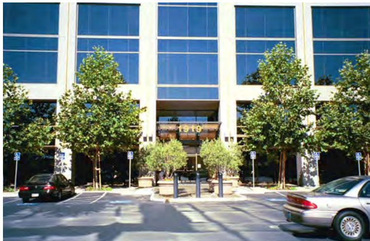
Pruneyard Towers- Campbell, CA
